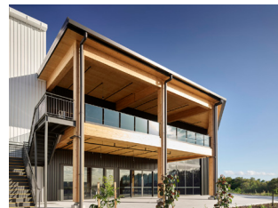
Industrial and Business Park Electrolux Group – Queensland Experience and Distribution Centre by Port of Brisbane
